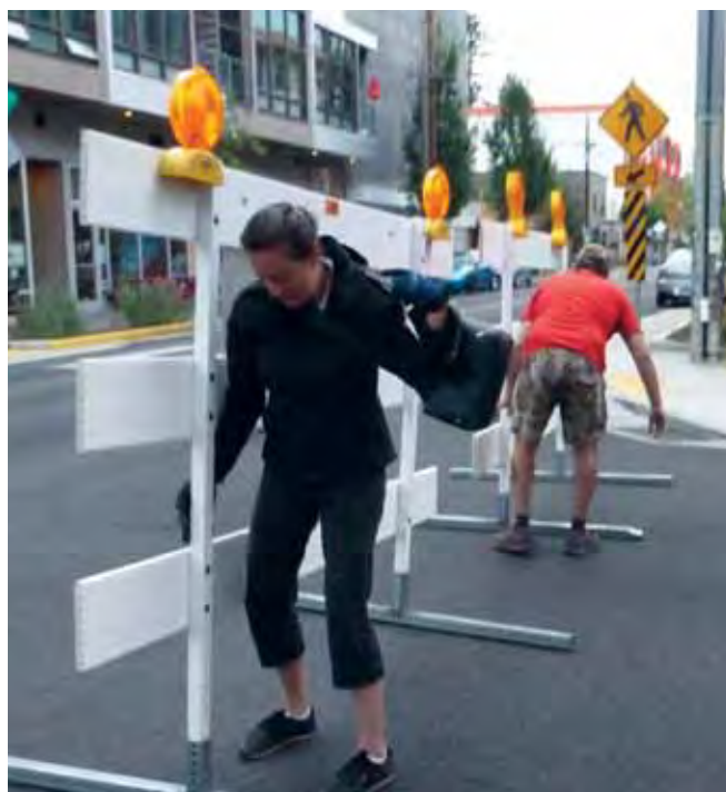
Teams of 2 work together when closing streets to save time and backs
